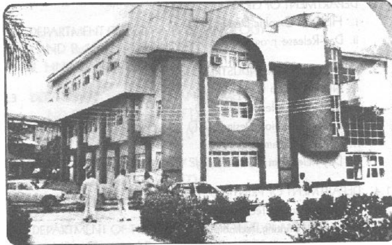
The newly commissioned School of Environmental Studies Building
